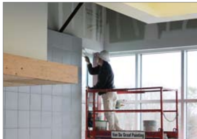
A painter primes the soffit in the double-height lobby.
