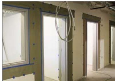
The old stairwell is now storage space and a shared office for band and chorus teachers adjacent to the new classrooms.
