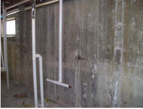
View of exposed concrete wall system in Laboratory Area (Adult Ed)
