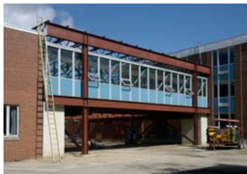
Structural steel is erected for a new music wing.
