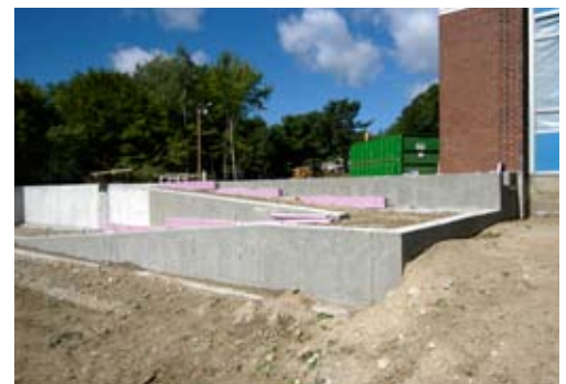
Foundations are in place for the new library and administrative wing.
