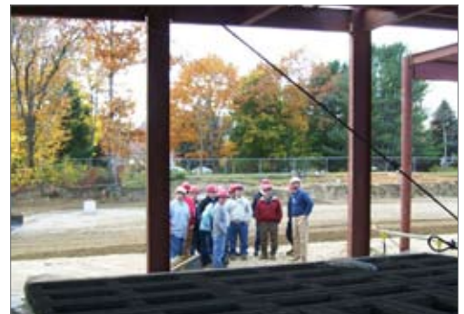
Students from the welding and metal fabrication class take a tour with Clerk of the Works Steve Drane to view the new steel.
