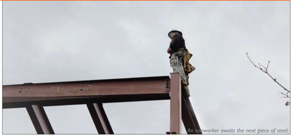
An ironworker awaits the next piece of steel.
