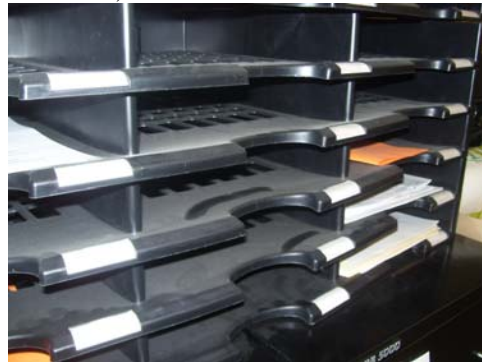
Room 222 – accumulated dust on file sorting trays (top of file cabinet)
